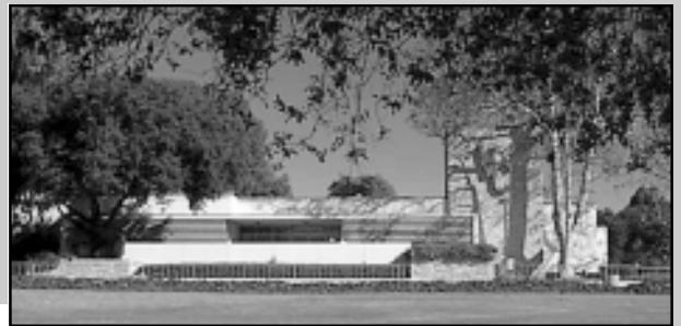
The project will improve instructional resources in the Ventura community.
